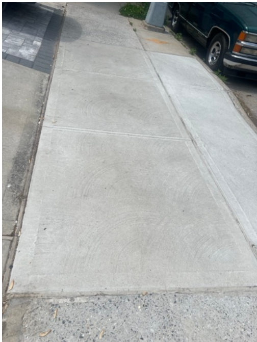
Sidewalk Material Concrete.
